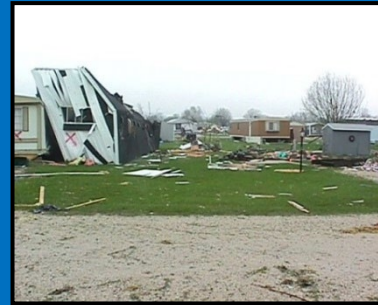
Significant Property damage
